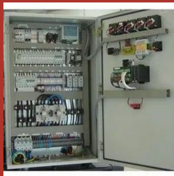
Panel Box Fabrication
